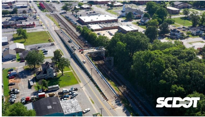
Image 1 Gaffney T-Bridge under construction
