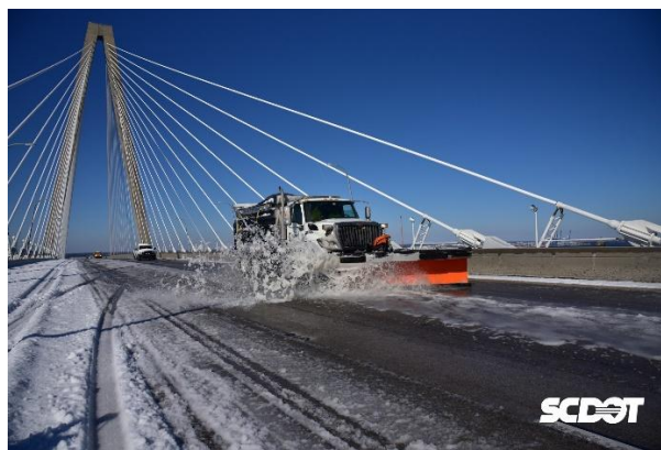
Image 5 SCDOT clears the Ravenel Bridge in Charleston
