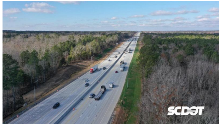
Image 2 Midlands Connection Project on I-26
